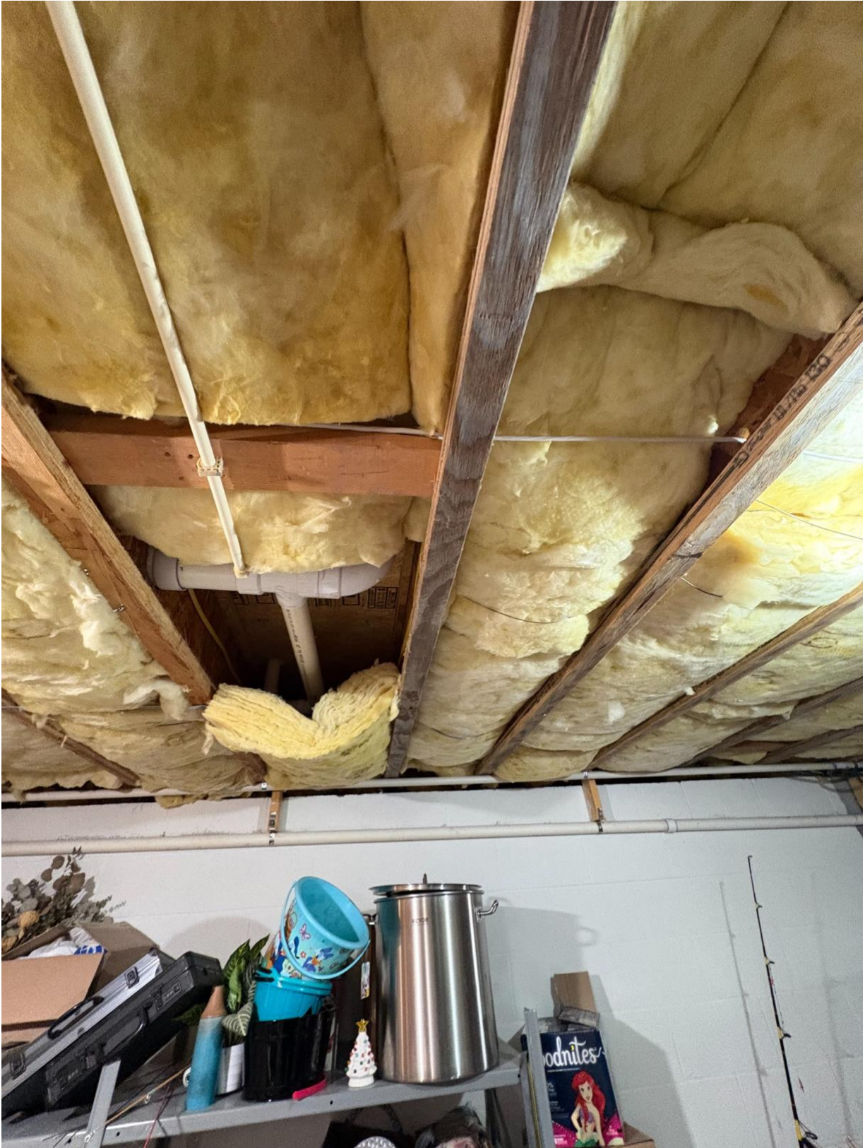
Photo 1 - Example overview of basement floor-joist bottoms and fiberglass insulation in the unfinished basement.
